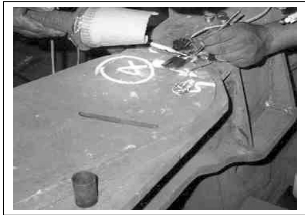
Fig 16 Strain gauge installation in the bogie
